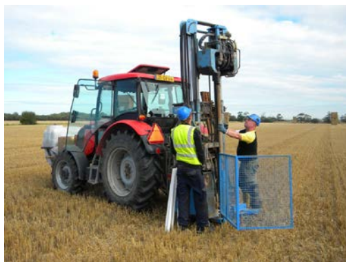
Tractor Mounted Drilling Rig
